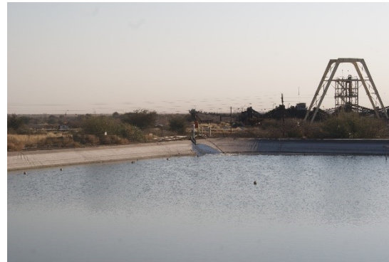
Sewage water being pumped into the return water dam
