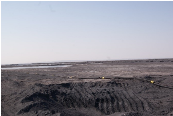
Top of slimes dam (almost full) with barge
