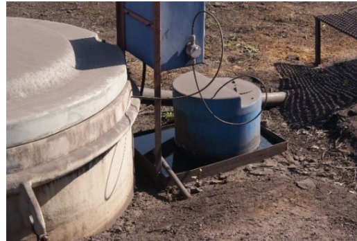
Broken chlorinator
