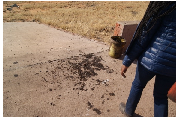
Hydrocarbon contaminated soil spillage at back entrance which is not trenched
