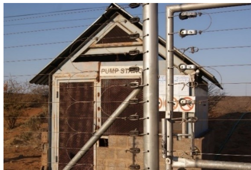
Adequate security access control
