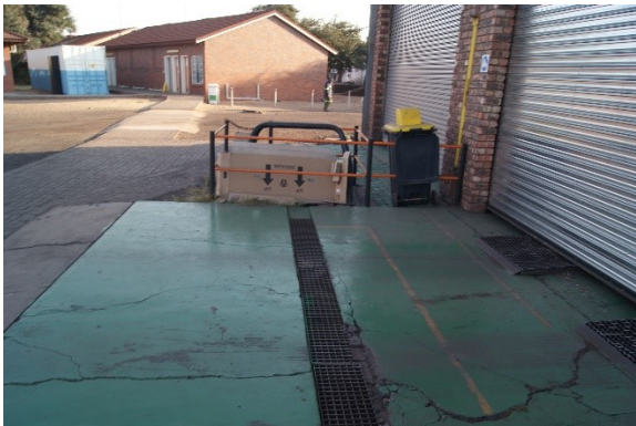
Secondary containment outside of workshop
