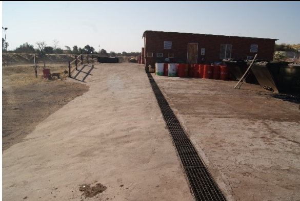
Bins and skips outside of the hazardous waste storage area on open ground
