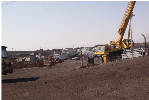
Temporary contractor area
