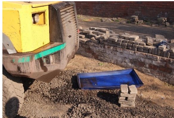
Hydrocarbon spills & drip tray
