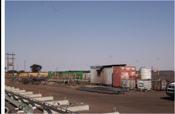
Contractor area next to old slimes dam
