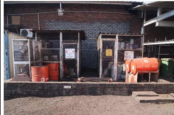
Chemicals stored outside of workshop were in a bunded area
