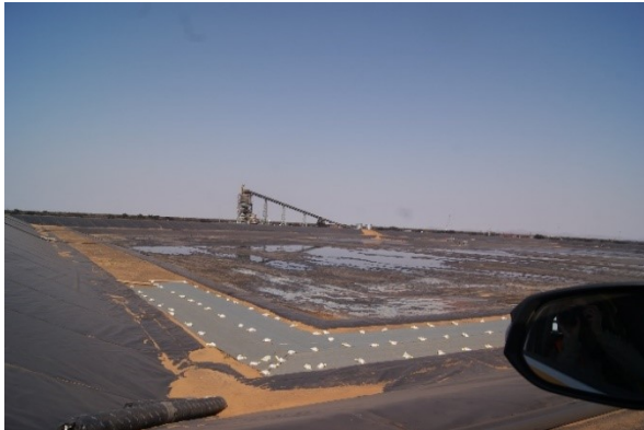
Top of slimes dam (almost full) with barge
