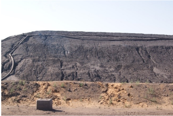
Old slimes dam's steep slopes
