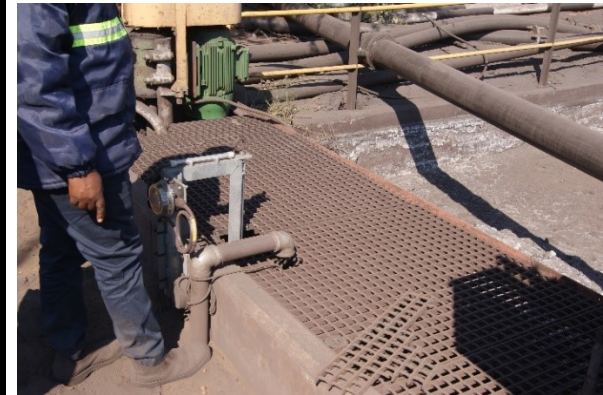
Silt trap to the return water dam not working
