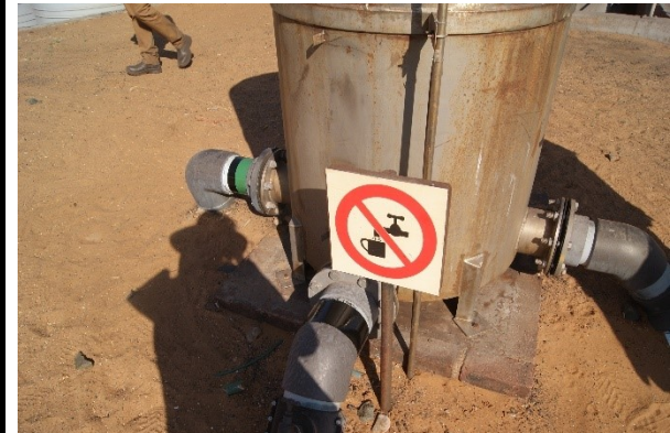
Colour coding on pipes to indicate chlorine
