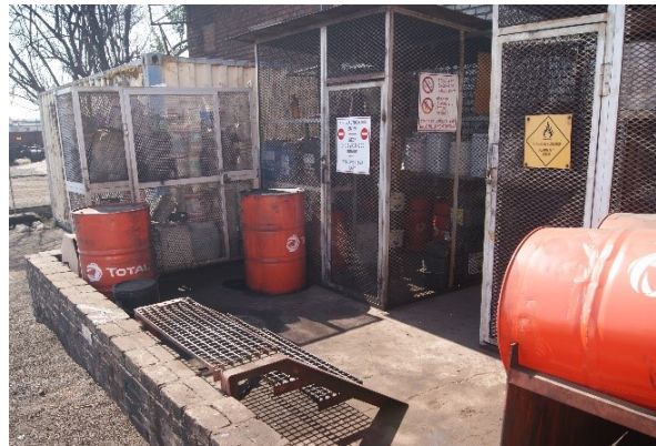
Chemicals stored outside of workshop were in a bunded area
