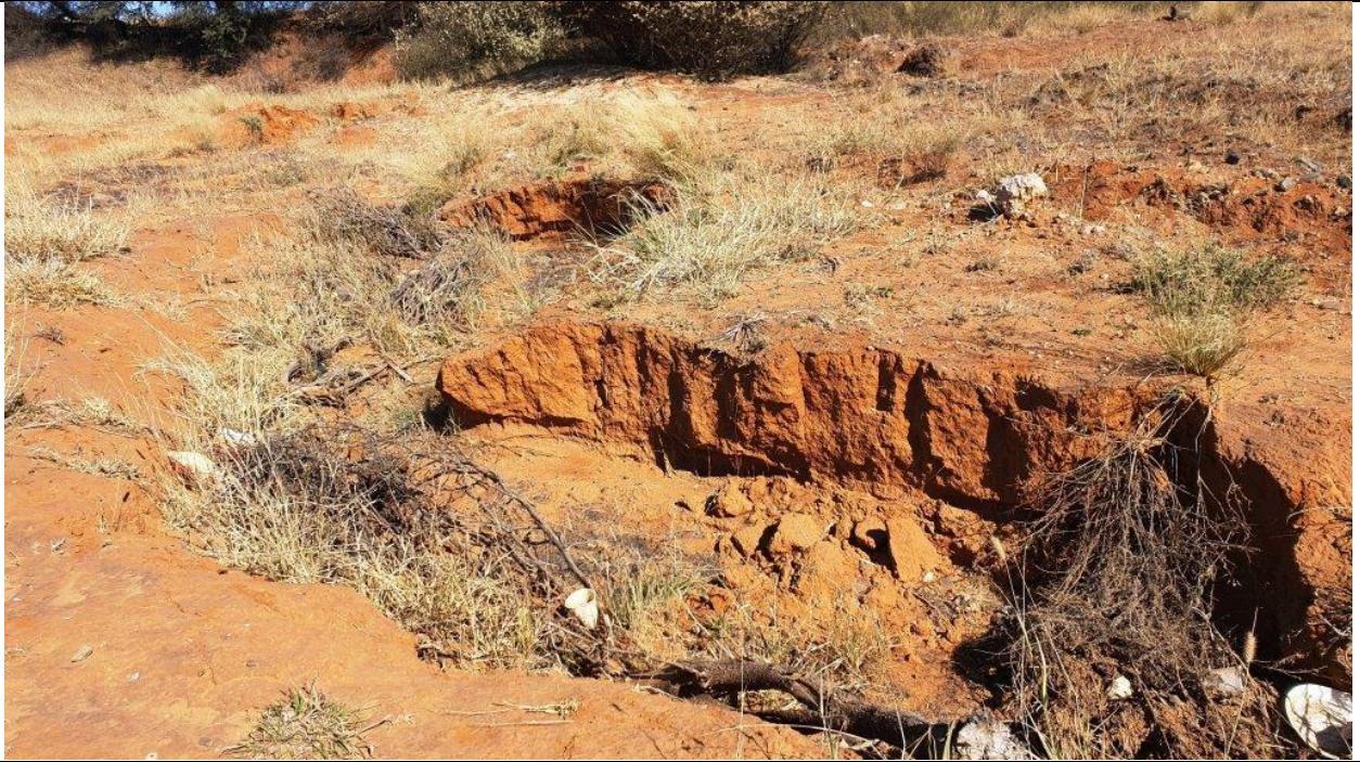
Figure 6.3: Erosion in rehabilitated area on Gamagara riverbank 3
