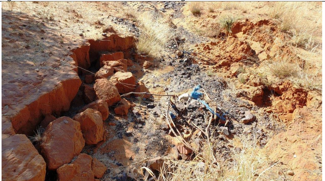
Figure 6.2: Erosion in rehabilitated area on Gamagara riverbank 2
