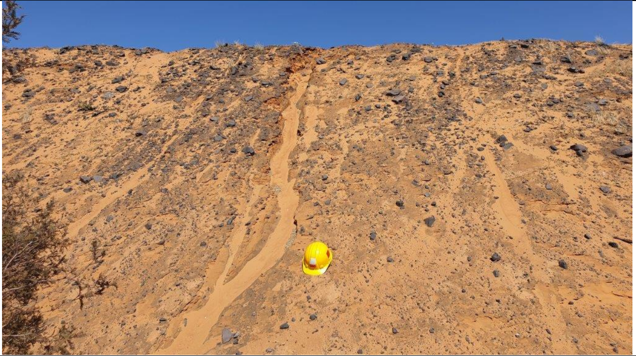
Figure 6.5: Erosion outside at Nchwaning 2 subsoil stockpiles from construction of the new TSF.
