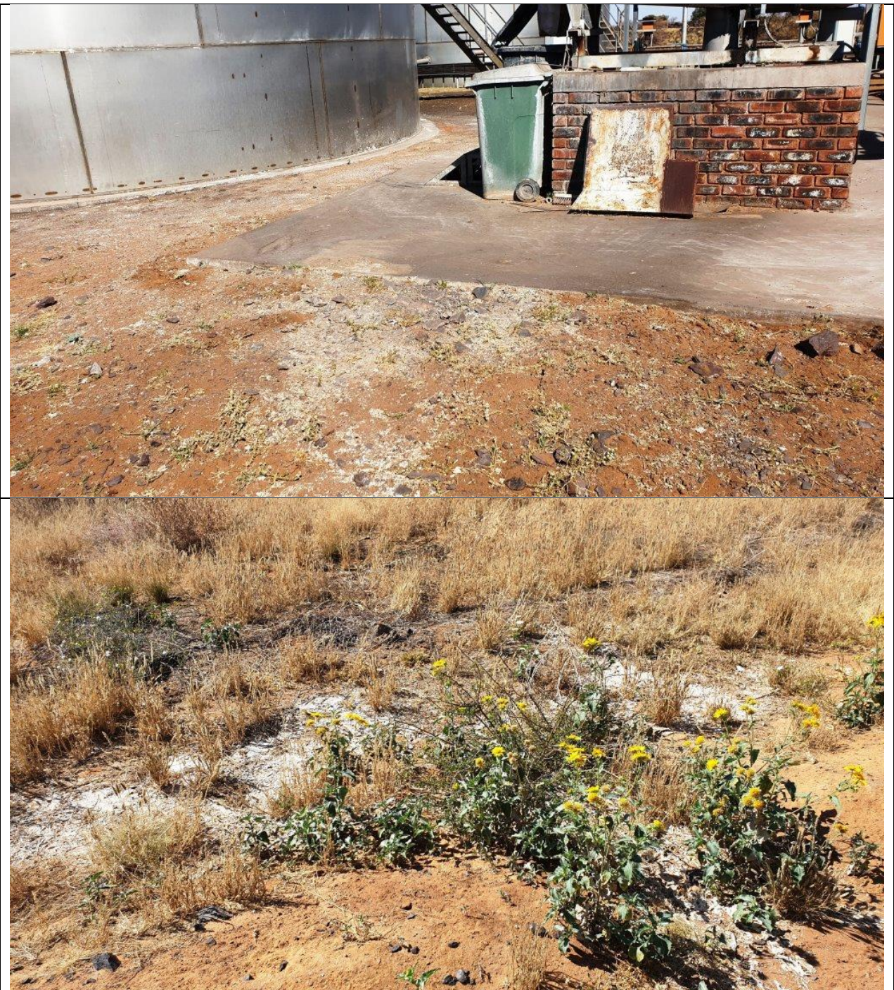
Figure 6.11: Overflows from at Black Rock Sewage Treatment Plant
