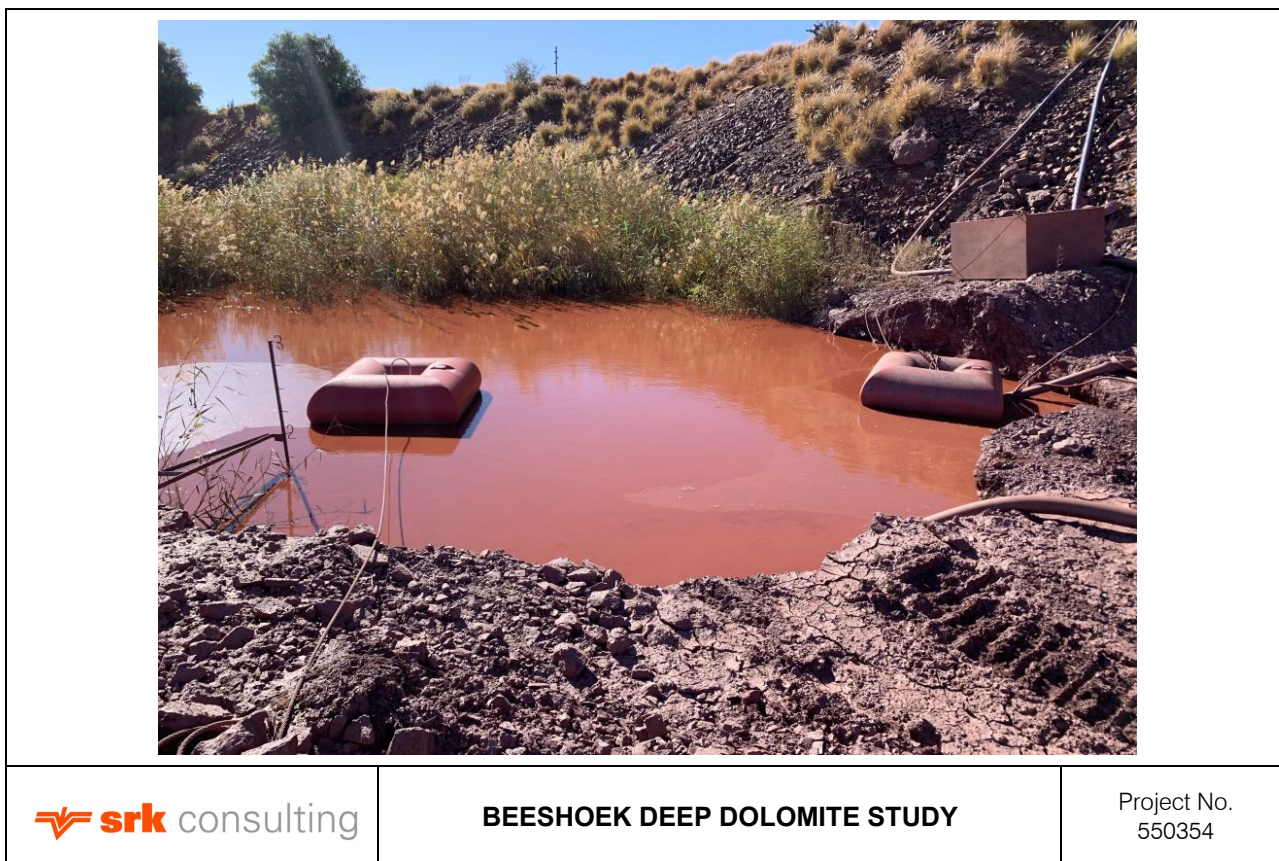
Figure 6-5 Supernatant pond adjacent to TSF embankment
