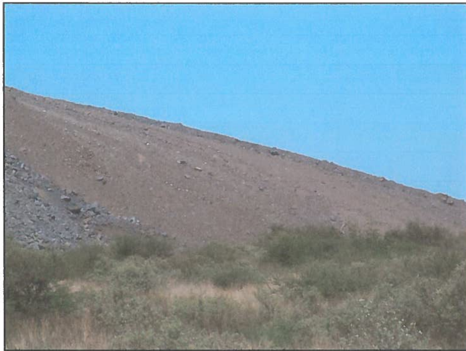
Figure 2: Beeshoek Iron Ore Mine Dumps sloped to 18°
