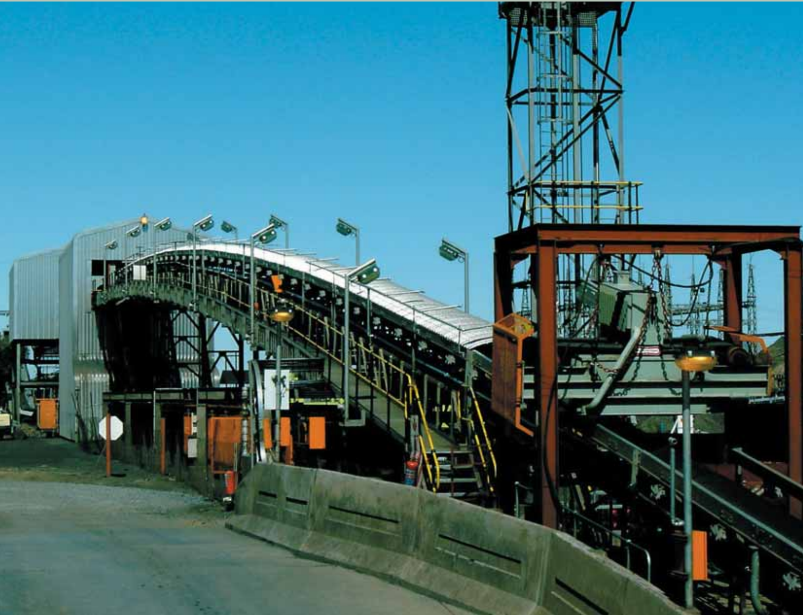
Nchwaning III conveyor
